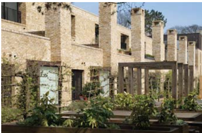
Countryside's Accordia, which organizes apartments and condos around productive gardens and connects them with footpaths and cycleways, was the first residential scheme to win RIBA's prestigious Stirling Prize in 2008.
